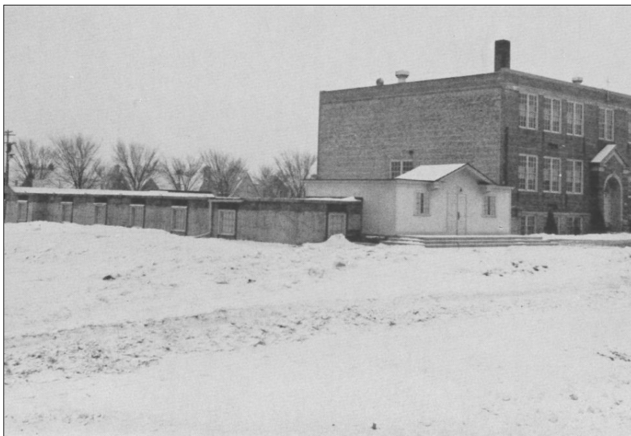
Exterior View of Basement Chapel
