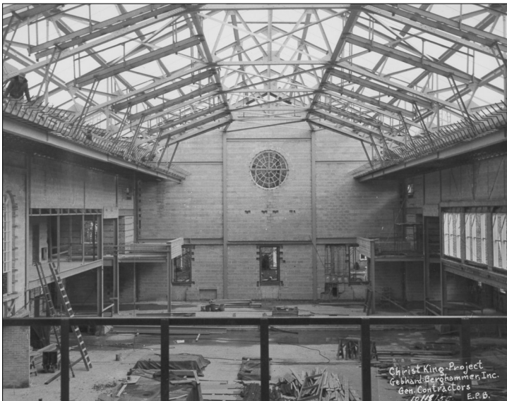
Church under Construction: October 1955
